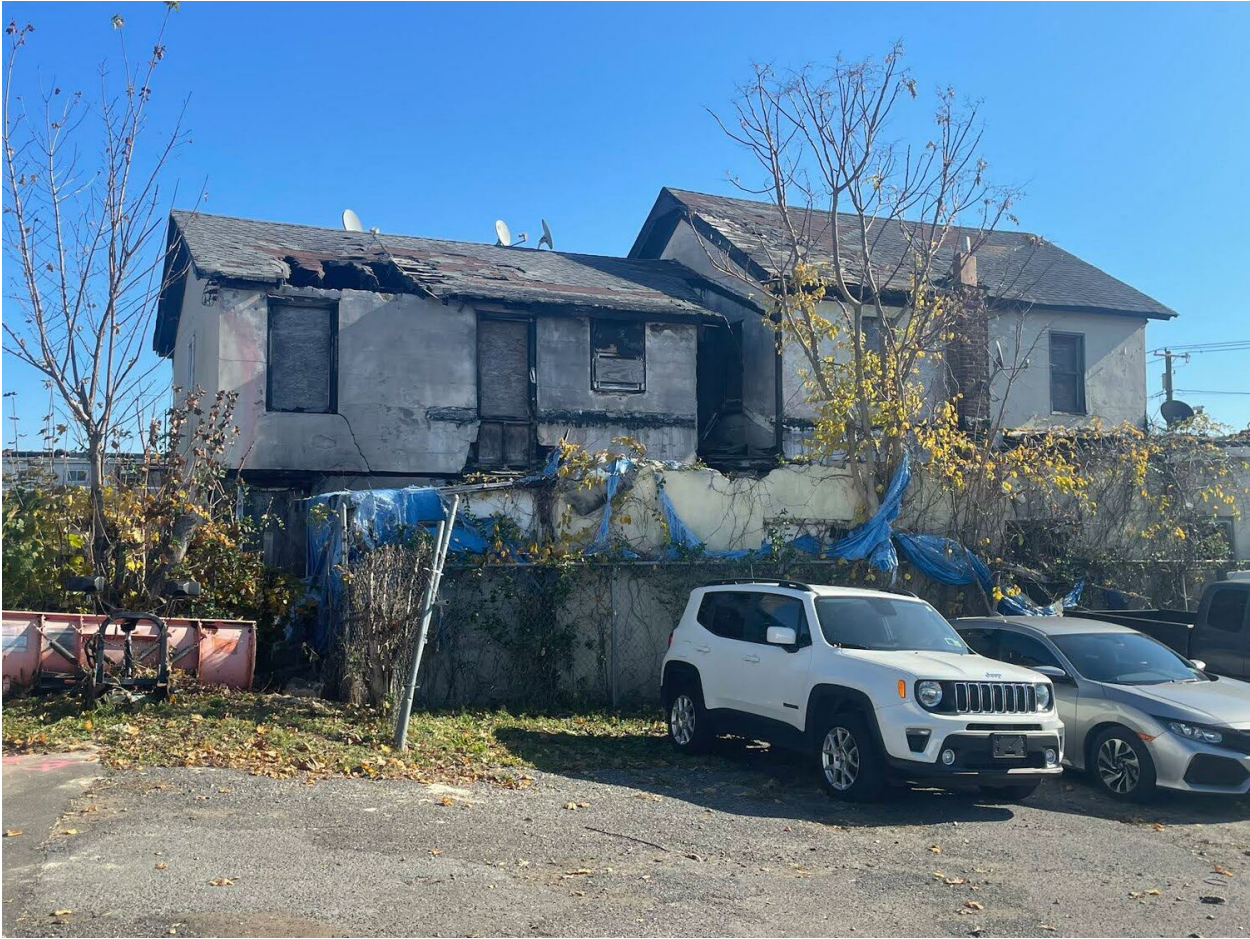
A view of the rear buildings that suffered from a fire
